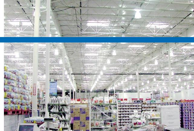
Ceiling temperature does not affect the excellent light output in this high bay application utilizing Venture's electronic Uni-Form® pulse start technology.
