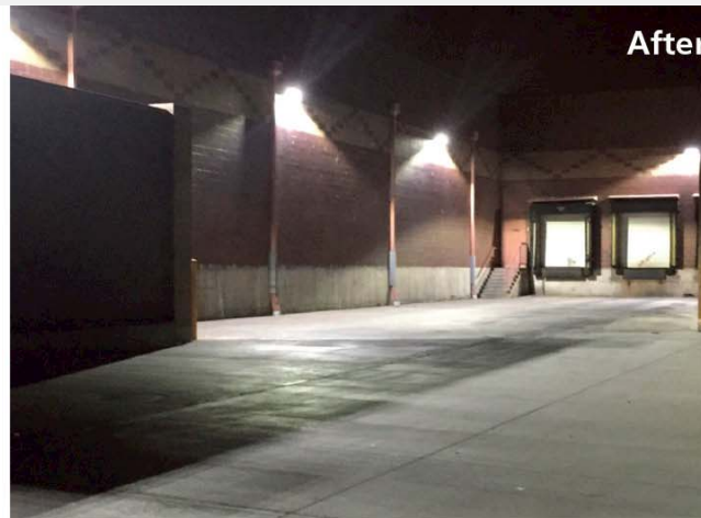
Shopping Center Receiving Area 400W MH Retrofitted with 81W LED wallpacks
