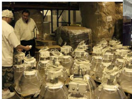
Liberty Lighting with Preferred Freezer during installation
